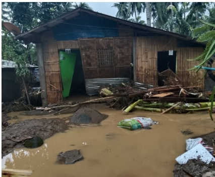
Homes Left Damaged and Unsafe
