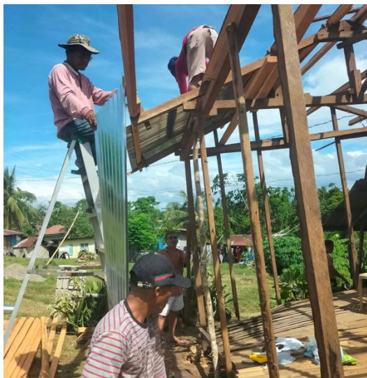
Rebuilding and Restoration
